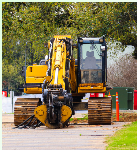
Photo by Alyus Dick Our Lady of Wisdom Church construction
