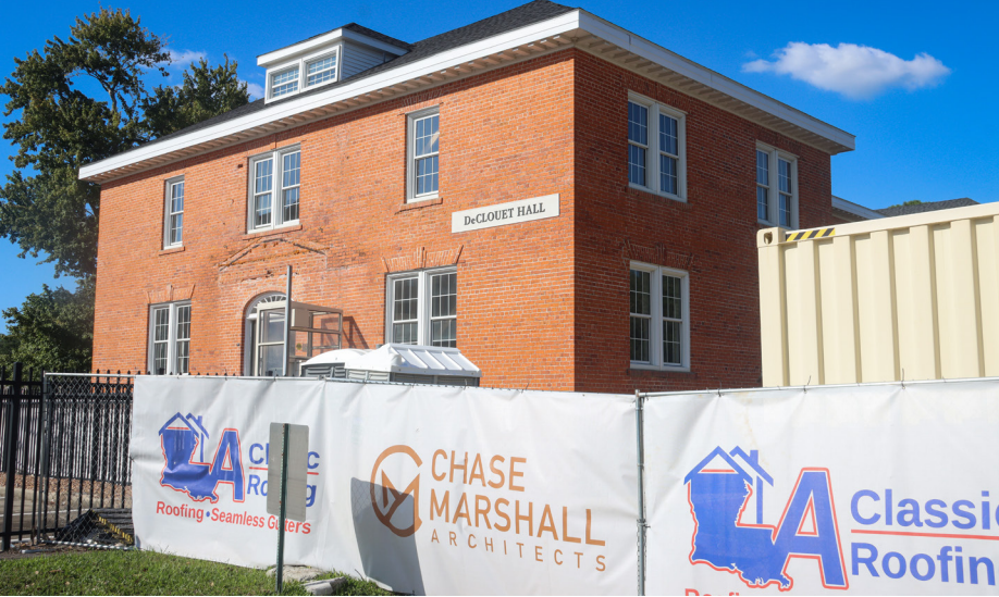
Photo by Alyus Dick Current construction site around DeClouet Hall
